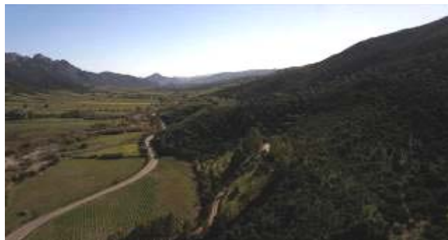
NUOVA S.S. 125 "ORIENTALE SARDA" 1° LOTTO CONSTRUCTION OF A NEW HIGHWAY CALLED "ORIENTALE SARDA"
